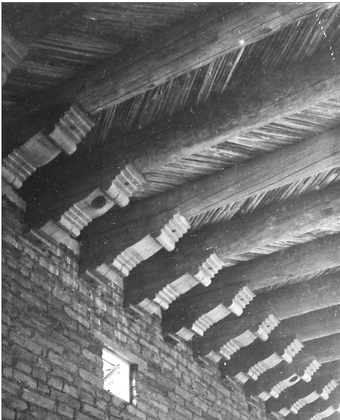
Figure 17. St. Michael and All Angels Episcopal Church, portion of nave ceiling during construction, 1953 (on file, Parish Office, St. Michael and All Angels Episcopal Church, Tucson; photographer unknown).
